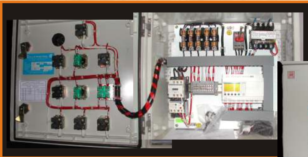
Grind Hog™ Controller Front & Inside Panel
