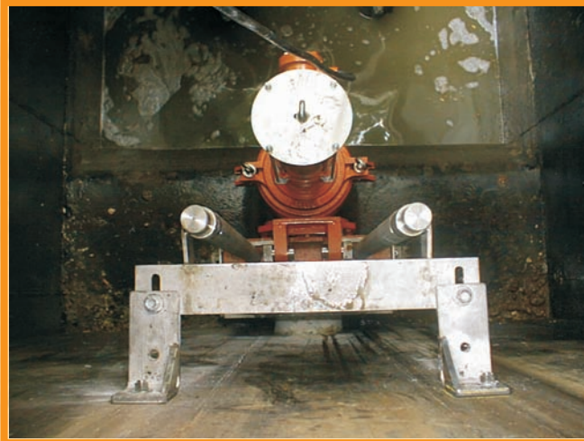
GRIND HOG TM 5AS A/C LOOKING DOWN FIXED TO SLIDE RAIL SYSTEM
