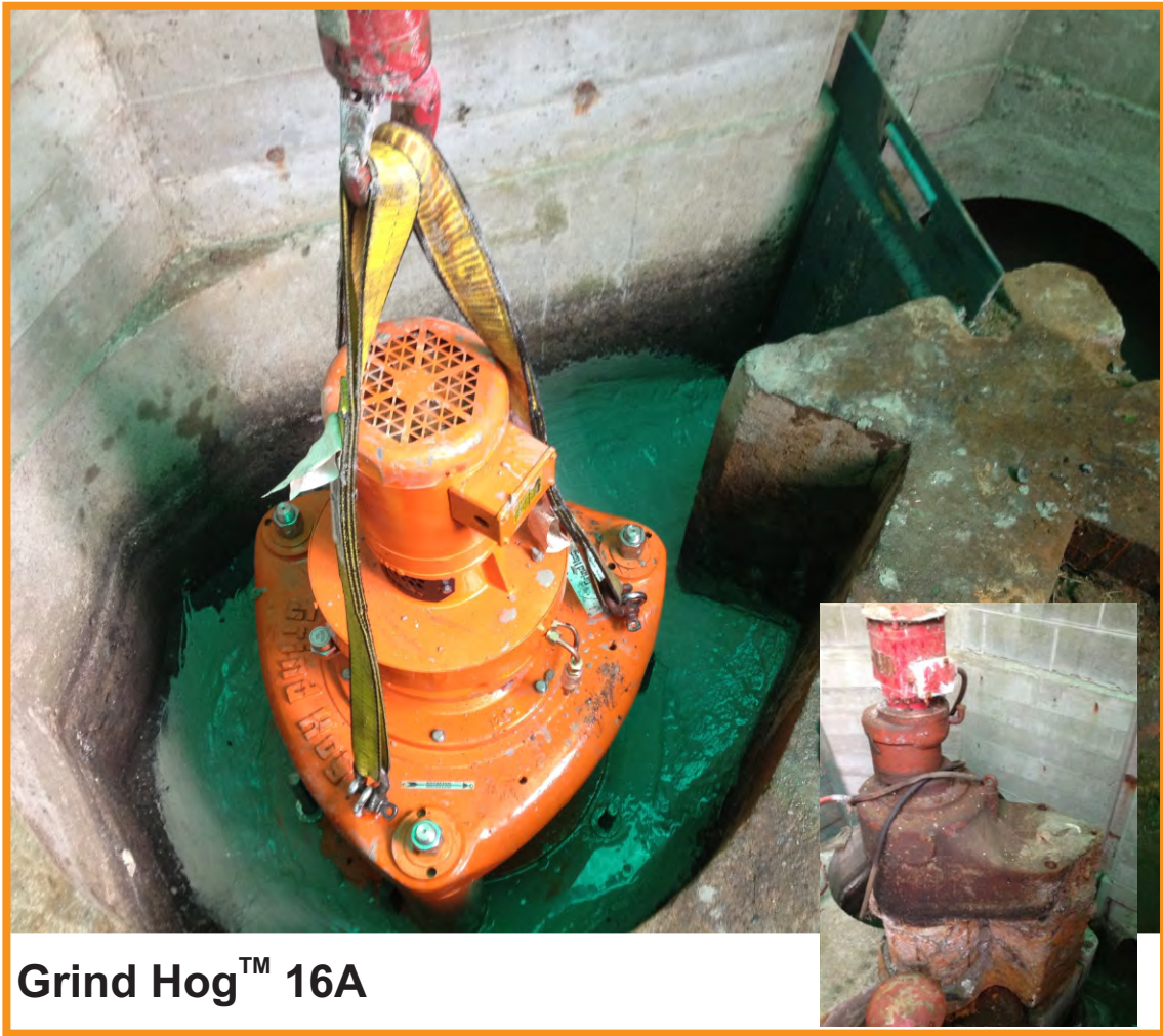
Previously Installed Jones & Attwood 15R (dimensionally similar to Chicago 15C)
